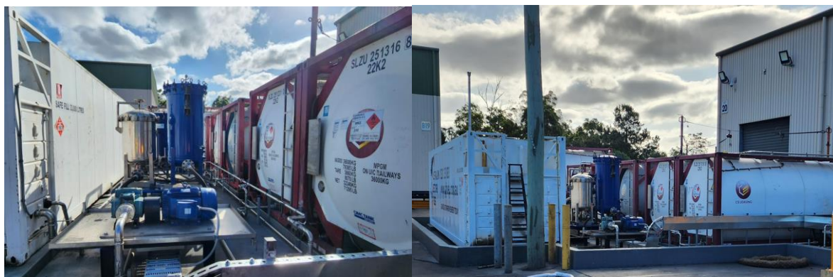
Image 3 and 4: Fuel management system installation on site at Stapylton: Source Company
