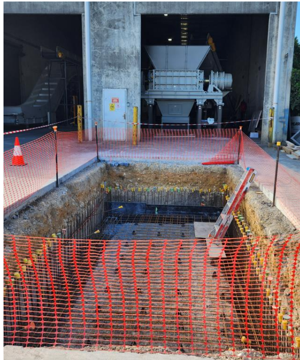
Shredding System being installed
