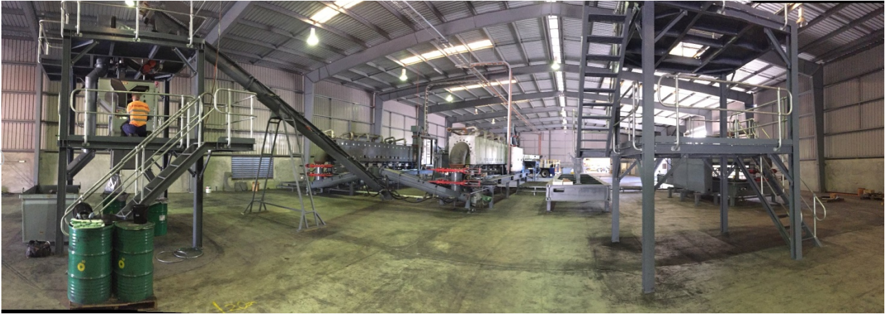
Photo courtesy of Pearl Global; Production Plant – Staplyton QLD.
