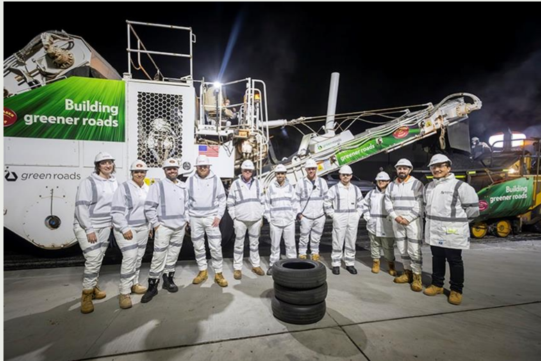
Pound road – road trial photograph courtesy Seymore Whyte & Alex Fraser
